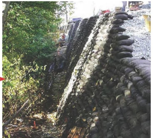
Deltalok V ® during Construction
